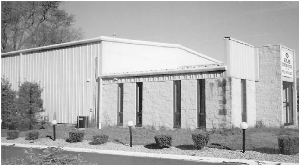
FIGURE 11.2 In this common design, a masonry front office abuts a pure metal building system in the back, raising concern about appropriate lateral drift criteria.
