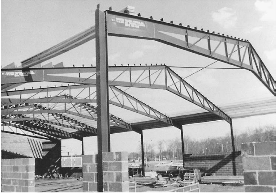
FIGURE 4.16 Trusses. ( Coronis Building Systems. )
