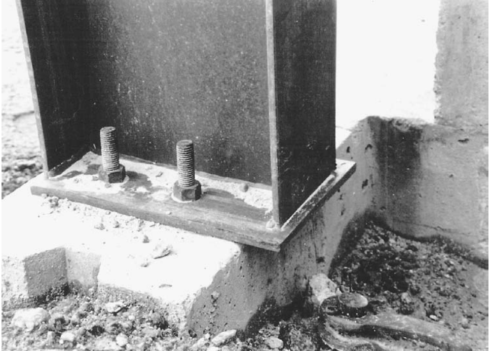
FIGURE 12.38 A column designed without regard to foundation size.
