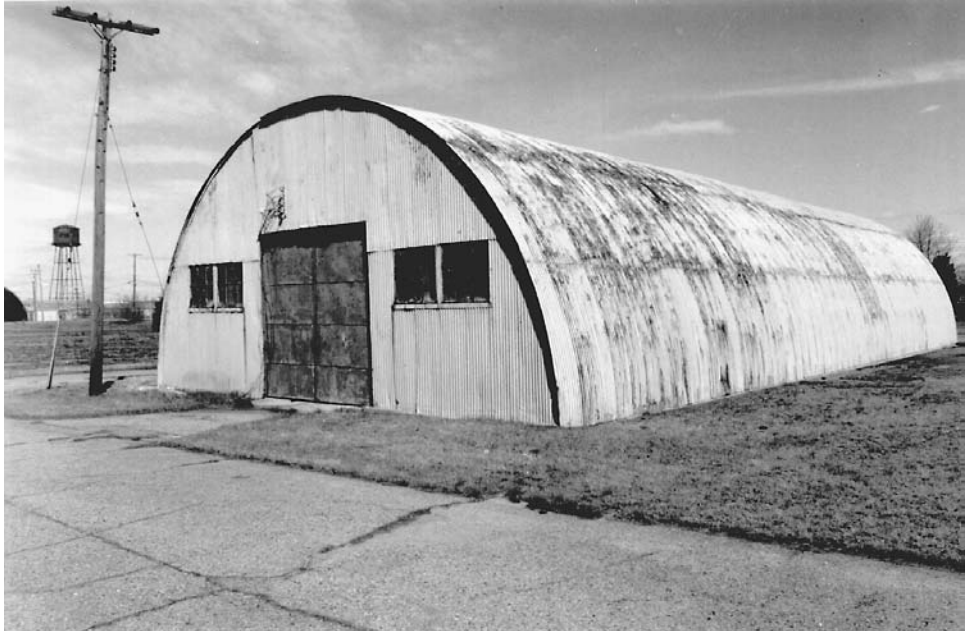
FIGURE 1.1 Quonset hut, Quonset Point, R.I. (Photo: David Nacci.)
