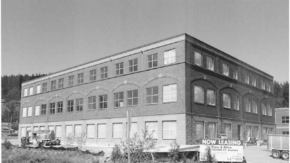
FIGURE 1.5 Office building of pre-engineered construction. ( HCI Steel Building Systems, Inc. )
