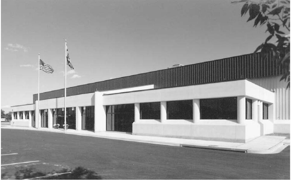
FIGURE 7.35 Precast wall panels add depth to the façade. (Photo: Maguire Group Inc.)
