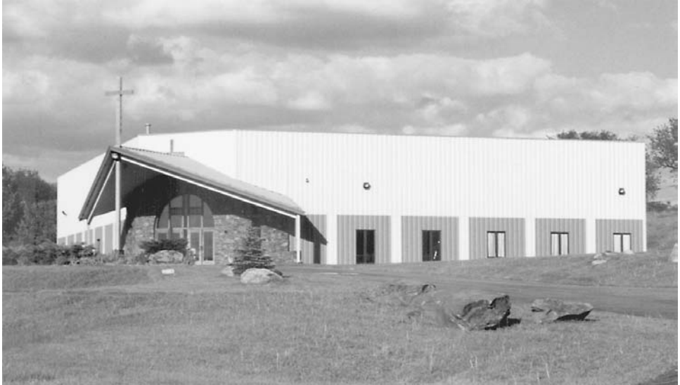
FIGURE 1.10 A church housed in a pre-engineered building.
