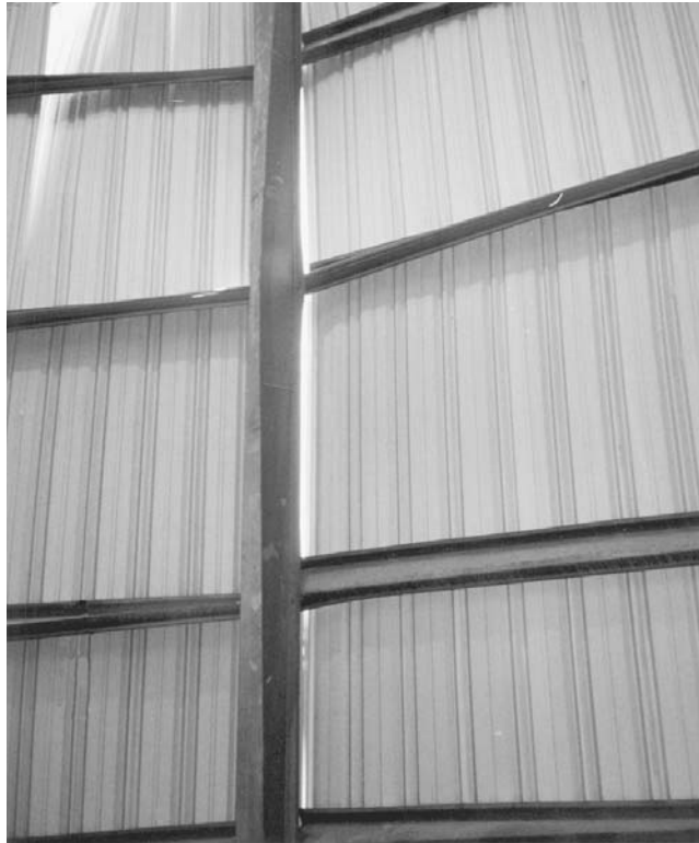
FIGURE 10.18 Buckling of laterally unbraced girts and endwall column under wind loading. (Photo: J.R. Miller & Associates.)
