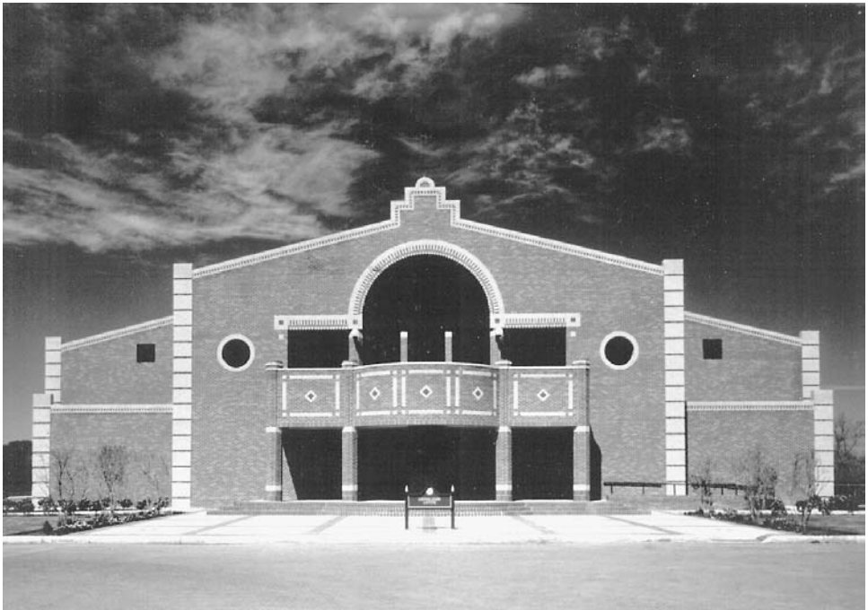
FIGURE 1.11 This community building utilizes a metal building system. (Photo: Metallic Building Systems.)
