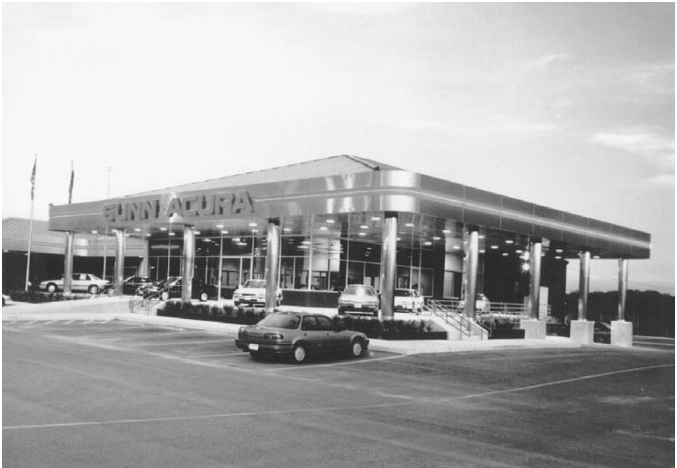
FIGURE 1.6 Auto dealership housed in a metal building. ( Photo: Metallic Building Systems. )
