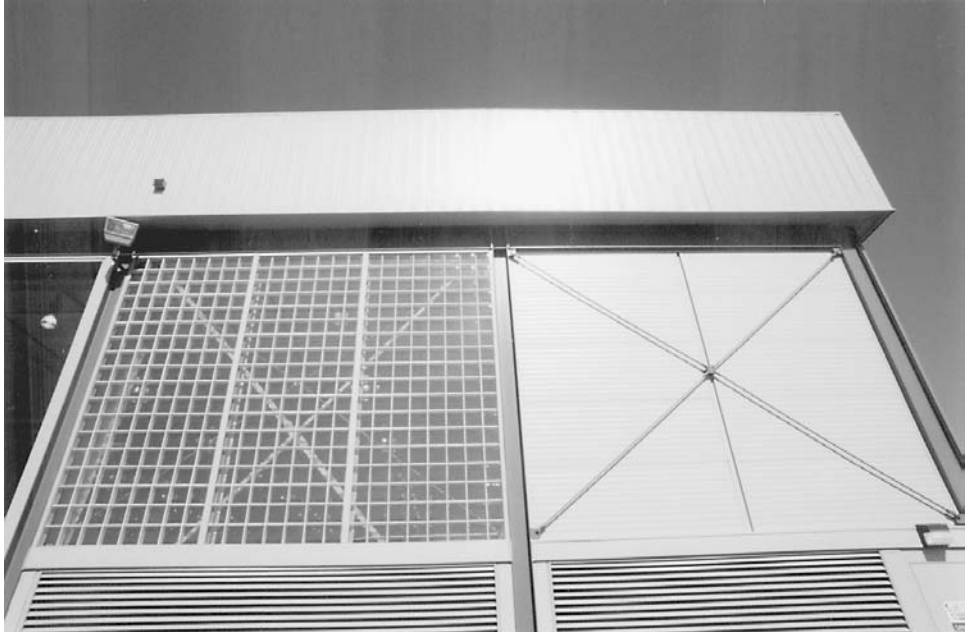
FIGURE 11.10 Presence of glass block in this metal building system justifies strict limits on building drift and racking. Note the interior wall bracing made of steel angles. (The exposed exterior bracing at right is purely cosmetic.) (Photo: Maguire Group Inc.)
